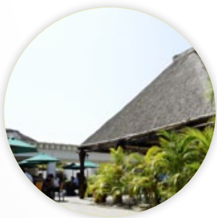
Traditional construction techniques are used at Huatulco Airport
